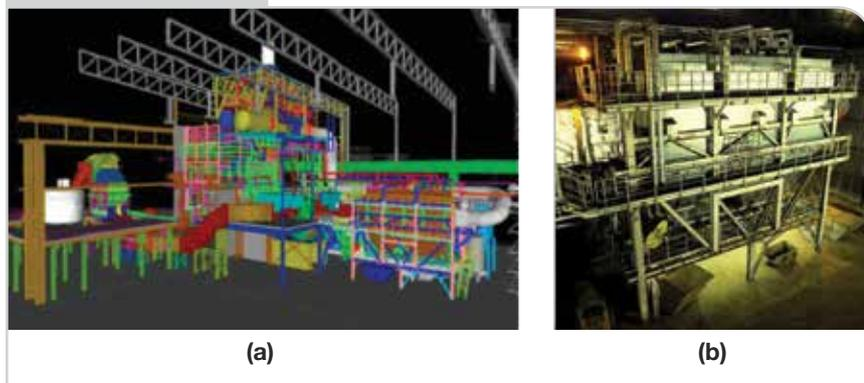
Waste heat steam generator rendering (a) and installed equipment (b) at ESF plant, Riesa.
