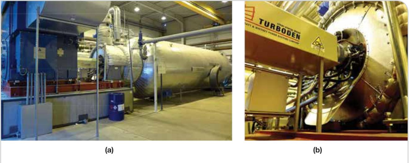
Organic Rankine cycle unit at ESF plant, Riesa: overview (a) and turbine detail (b).
